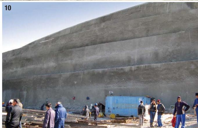
9- Gutter of clayey scree on a substratum of clayey schists of low resistance (earth cuts subsequently strengthened).
